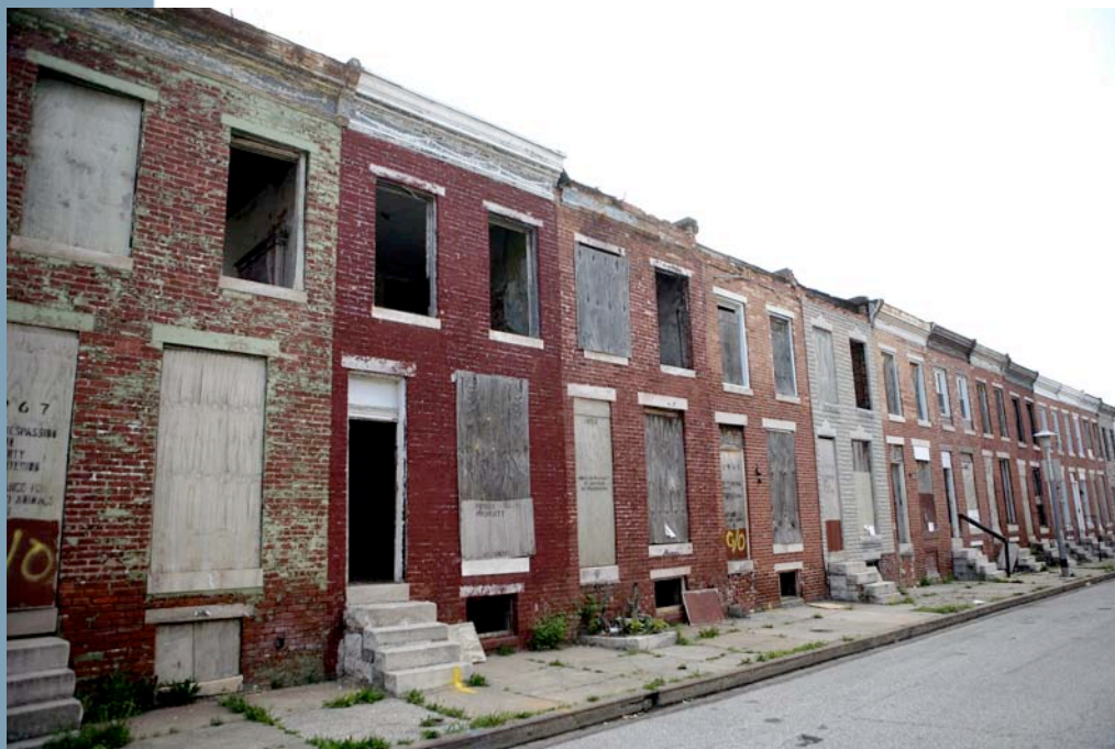
1900 Perlman Place -Recently demolished by Mayor Rawlings-Blake.
